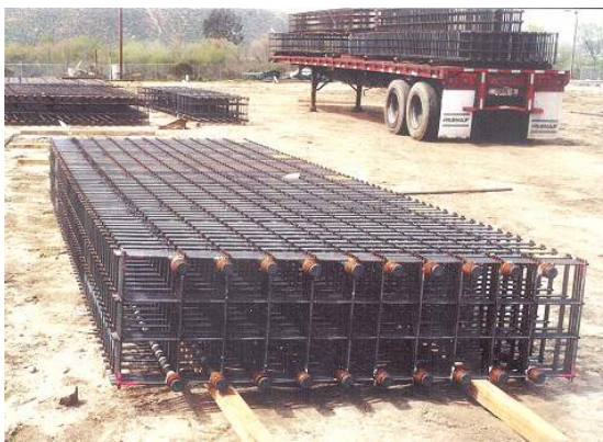
Figure 3 - Cage made with BauLadders, which, as shown, also ship very compactly
