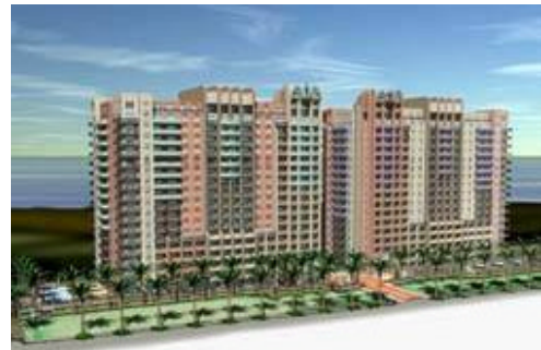
Figure 5 - Long Beach Project Showed 75% Cage Assembly Labor Reduction
