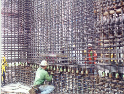
Figure 8 – Rapid Installation of BauGrid® WRG Cages Using SpliceGrids™
